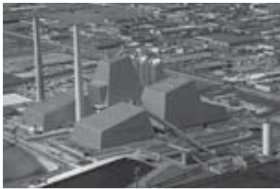
Avedøre thermal power plant No.1 and No.2 of ENERGI E2 Co. in Denmark
